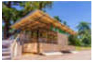
OFF BAR Florence 2014 | ND Studio: The structure is designed using metal scaffolding tubes and wooden pallets originally intended for transporting goods. The solution is easy to assemble and has a simple form, making it versatile and customizable according to the client's needs.
